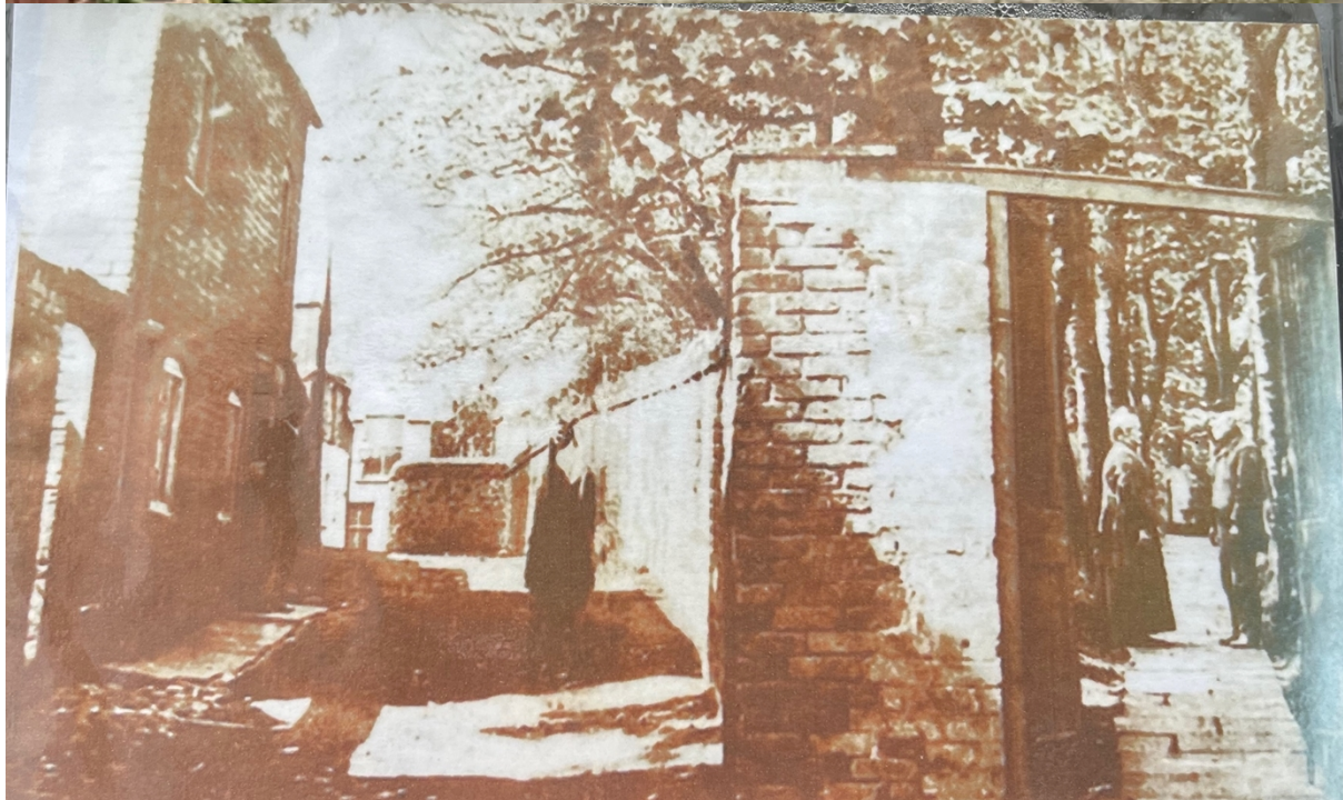
Undated photograph of route under investigation on display on notice board looking back up the route from point C [above]
